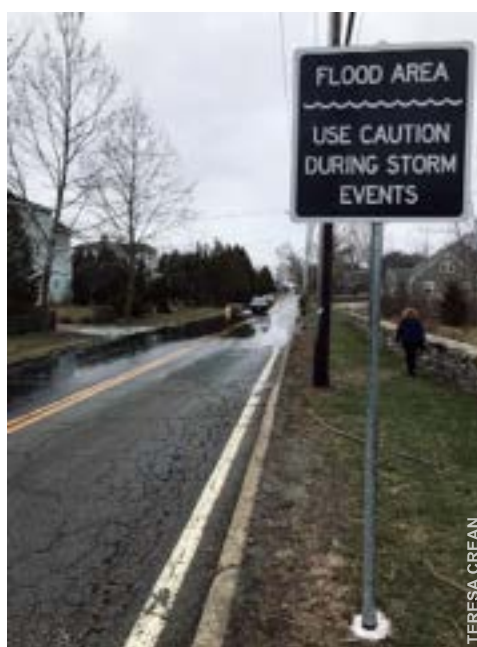
Segments of Rhode Island's road network are exposed to high tides and storm surge flooding; they will be further compromised by rising seas in 2050.
