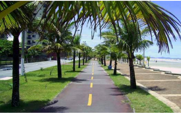
A waterfront bikepath running adjacent to traffic
