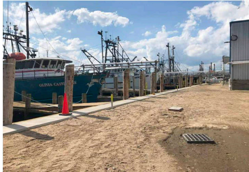
Dockside renovations within the port
