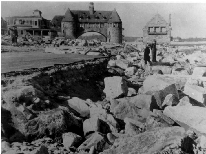
Storm damage to Coastguard House in Narragansett
