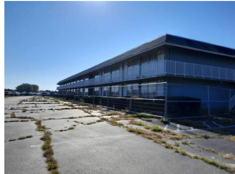
Back view of the property, northeast corner.
