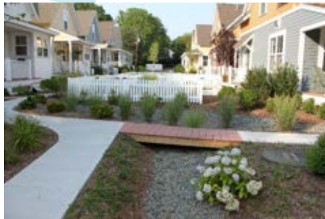
Cottages on Greene - bioretention, bioswales, and permeable pavement in compact cottage development in East Greenwich.
