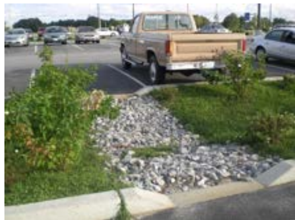
Bio-infiltration swale at a commercial parking lot in North Kingston. The curb cut allows stormwater to enter the system.
