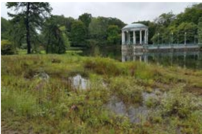
Roosevelt Lake Recreational Path is comprised of a rain garden, bioswale and restored shoreline buffer in Roger Williams Park, Providence. These areas treat stormwater from nearby roads and parking lots and discourage geese.
