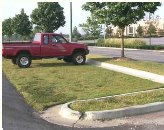
TOP RIGHT: Where site conditions allow, pervious options like this block paver driveway should be considered (Chesapeake Bay Program). LEFT: The pervious block paver onstreet parking lane on Broadway in Newport (S. Wheeler). CENTER: Reinforced turf overflow parking lot (Smart Growth / Smart Energy). RIGHT: Pervious asphalt parking spots on the right and conventional asphalt to the left at Cottages on Greene in East Greenwich (J. Ford).
