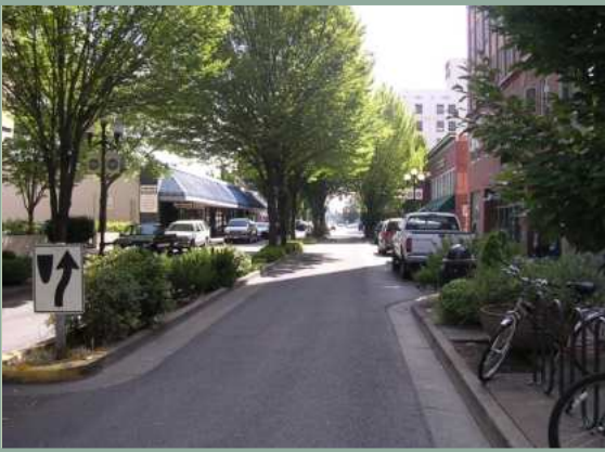
Bumpouts in sidewalks can be used to catch stormwater and to provide enough rooting space for trees as well as slowing traffic and creating safer crossing for pedestrians (NACTO).
