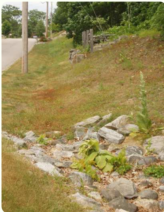
LEFT: Open-section grassed swale in North Kingston. CENTER TOP: Infiltration trenches on each side of the road in North Kingstown recharge groundwater. CENTER BOTTOM: A grassed swale in a Massachusetts development planted with turf and clover (MASS Smart Guide Toolkit). RIGHT: Stormwater can move between the open-section swales on either side of this driveway in the low impact development Jordan's Cove, Connecticut (CT NEMO).
