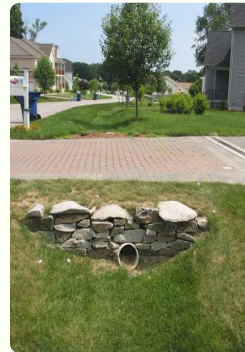
LEFT: Open-section grassed swale in North Kingston. CENTER TOP: Infiltration trenches on each side of the road in North Kingstown recharge groundwater. CENTER BOTTOM: A grassed swale in a Massachusetts development planted with turf and clover (MASS Smart Guide Toolkit). RIGHT: Stormwater can move between the open-section swales on either side of this driveway in the low impact development Jordan's Cove, Connecticut (CT NEMO).
