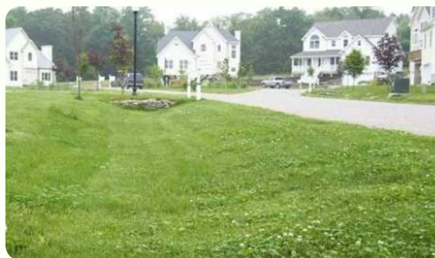
LEFT: Open-section grassed swale in North Kingston. CENTER TOP: Infiltration trenches on each side of the road in North Kingstown recharge groundwater. CENTER BOTTOM: A grassed swale in a Massachusetts development planted with turf and clover (MASS Smart Guide Toolkit). RIGHT: Stormwater can move between the open-section swales on either side of this driveway in the low impact development Jordan's Cove, Connecticut (CT NEMO).
