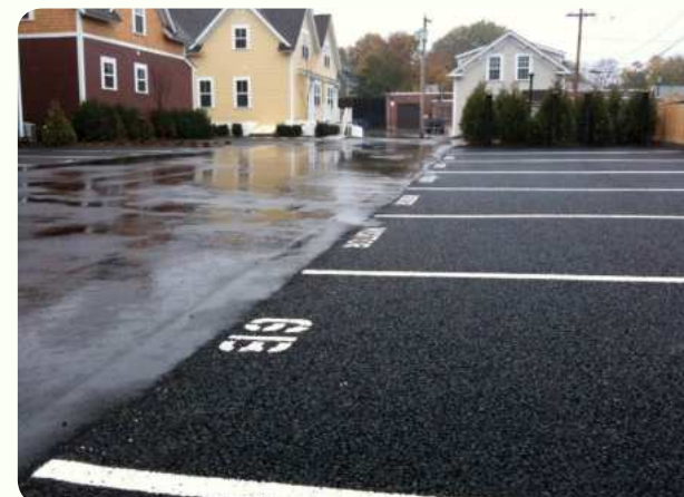
TOP RIGHT: Where site conditions allow, pervious options like this block paver driveway should be considered (Chesapeake Bay Program). LEFT: The pervious block paver onstreet parking lane on Broadway in Newport (S. Wheeler). CENTER: Reinforced turf overflow parking lot (Smart Growth / Smart Energy). RIGHT: Pervious asphalt parking spots on the right and conventional asphalt to the left at Cottages on Greene in East Greenwich (J. Ford).
