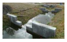
Outlet Control Structure: A hydraulic structure placed at the outlet of a channel, spillway, pond, etc., for the purpose of dissipating energy, providing a transition to the channel or pipe downstream, while achieving the discharge rates for specific designs
