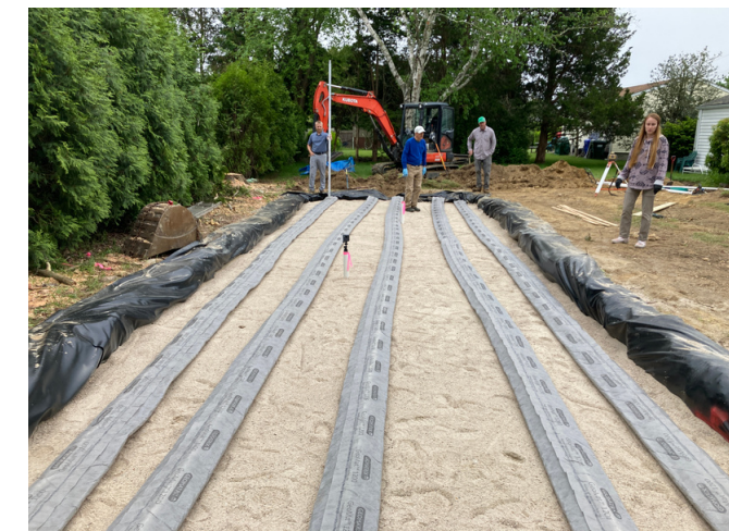
Installing an experimental nitrogen reducing drainfield system
