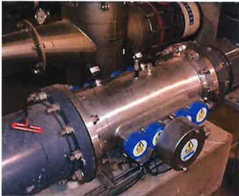
UV Unit install and repair
