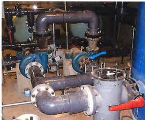
Pump and filtration work
