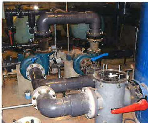
Pump and filtration work
