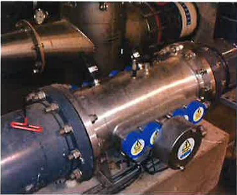
UV Unit install and repair
