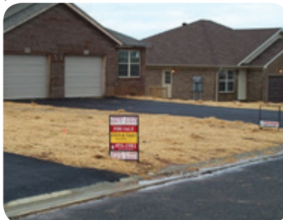
Straw mulching is a good way to prevent soil erosion. Photo credit: Barry Tinning at Tetra Tech.
