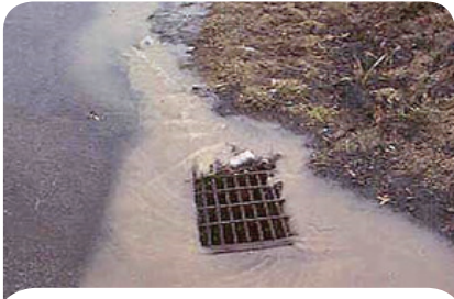
Muddy water flowing from construction sites is an illicit discharge.
