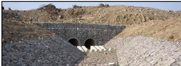
Gabion mattresses constructed to prevent erosion in an area of flow
