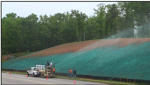
Hydroseeding a slope along a roadway to stabilize soils and prevent erosion
