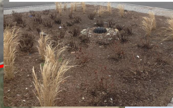
Runoff redirected to bioinfiltration area placed in former parking area
