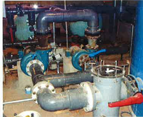
Pump and filtration work
