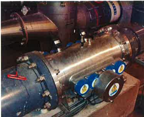
UV Unit install and repair
