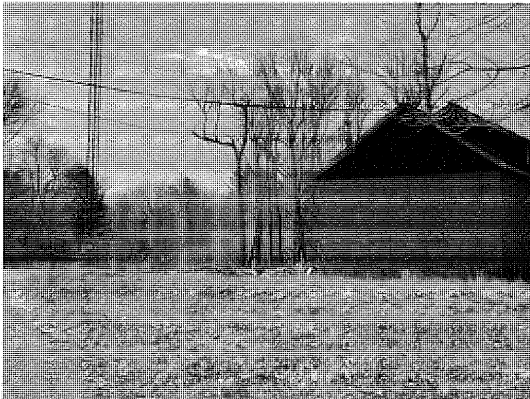
Photo 3 – URI Radio Tower Control Room
