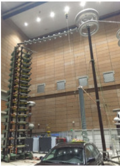
TU Darmstadt- High Voltage Lab
