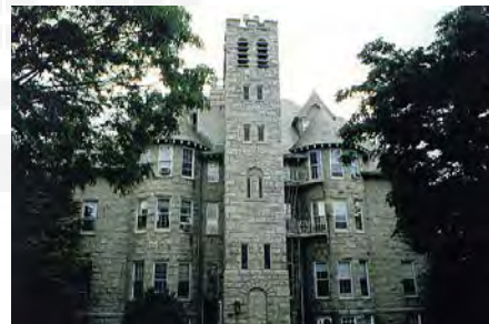
Relocating current uses out of Davis Hall would free up 12,600 NSF, which could be available for teaching programs.
