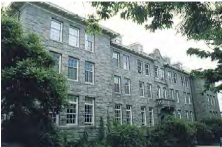
Historic Ranger Hall will be rehabilitated and available for reassignment.
