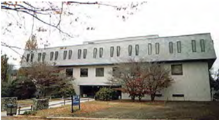
Renovations at Ballentine Hall will take 16 classrooms temporarily (and 4 permanently) off-line.
