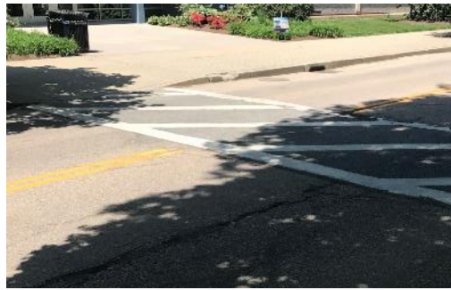
Diagonal crosswalk lines are not recommended because they are not as visible
