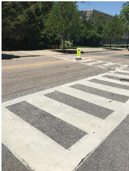
"Ladder" style crosswalk marking are recommended and consistent with Campus Design Standards
