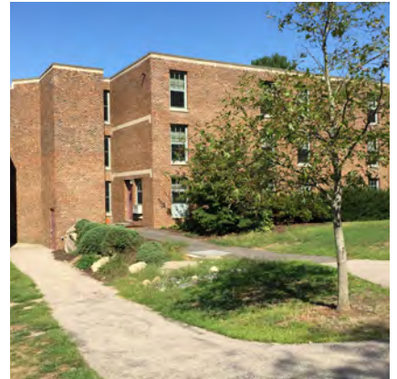
Slopes should require low maintenance, "no mow" vegetation
