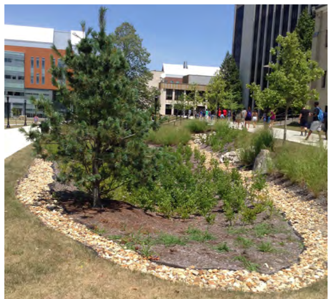
A newly installed bio-swale will help filter silt and pollution from surface runoff.
