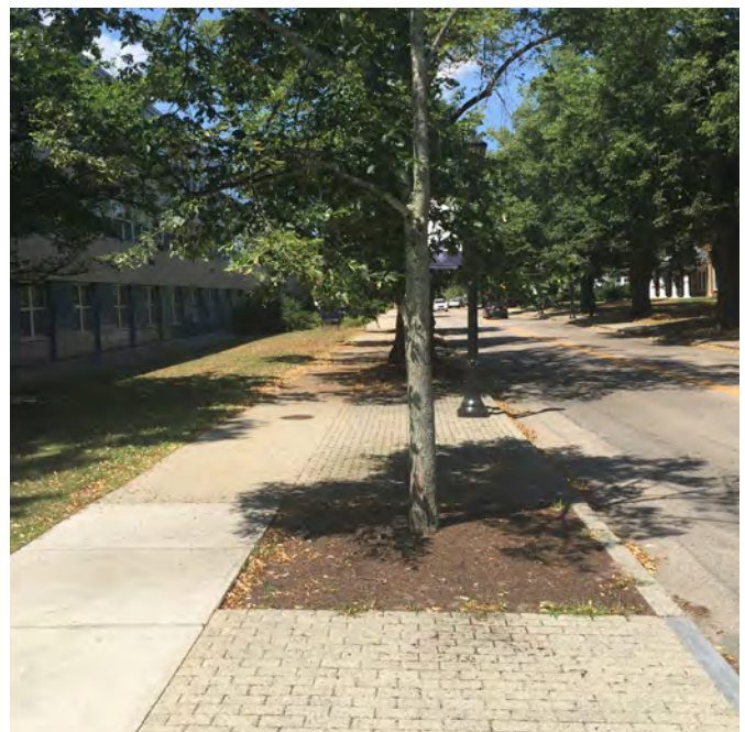
Tree planted in tree pit with pervious pavers (Upper College Road)
