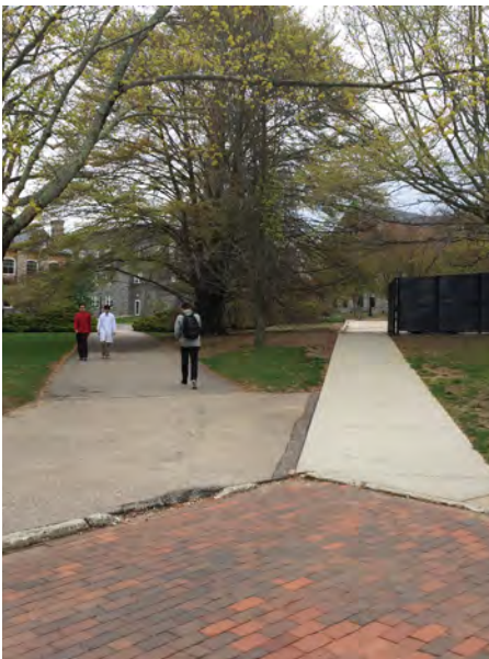
Curbs creating tripping hazards
