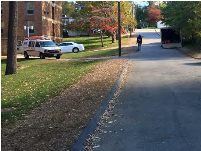
A lack of proper sidewalk caused pedestrians to walk on the edge of turf. This social trail and excessive use prohibits the growth of any turf.
