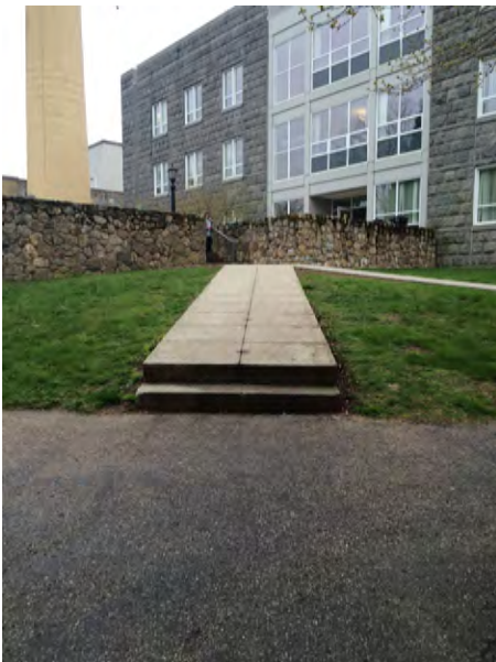
Poorly designed, sloped walkway
