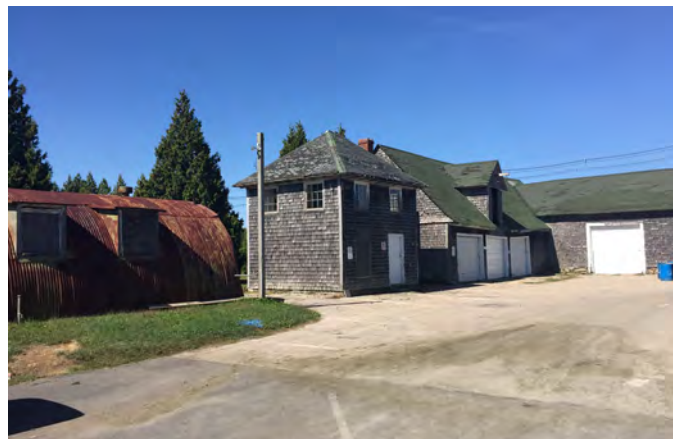
The athletic storage buildings are in need of replacement.
