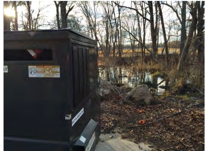
A dumpster is shown placed in close proximity to a wetland. This dumpster should be relocated away from areas that are sensitive to pollution.
