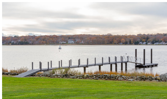
Dock off the western shore of the Touisset peninsula in Warren (Image from https://www.eastbayri.com/stories/this-dock-is-built-to-last,95592 )
