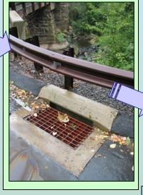
Catch basins are connected by pipes to other catch basins. picking up water from each basin as it travels through the system.
