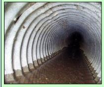
From the catch basin, the water enters a pipe. Catch basins are connected to each other by these pipes. The runoff travels down the pipes by gravity, flowing to the lowest point in the system, where the water exits the system.
