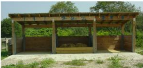
Aerated Bay Compost System. URI Peckham Farm, September 2010.
