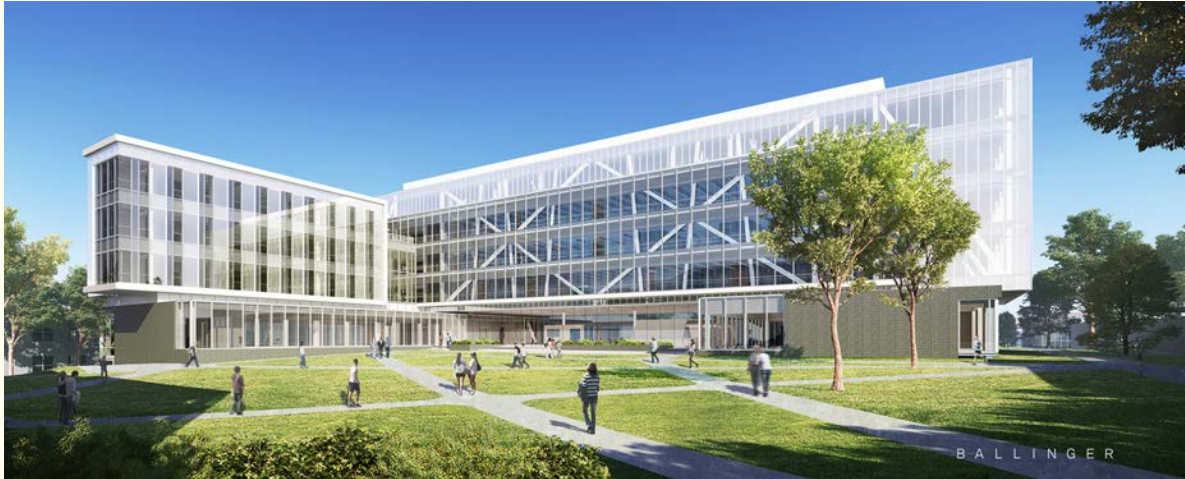
New College of Engineering Building
