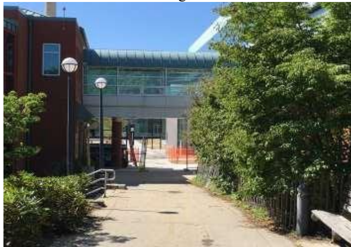
Photo 2: Kirk Building Pedestrian Overpass
