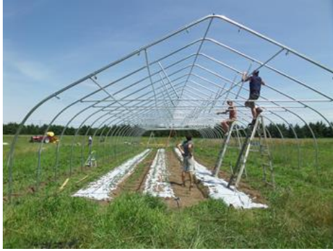
High tunnel under construction at Brandon Family Farm.
