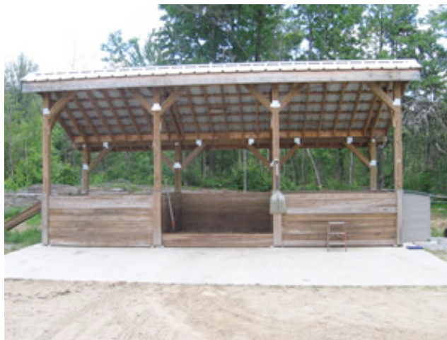
Roofed composting system on concrete pad.
