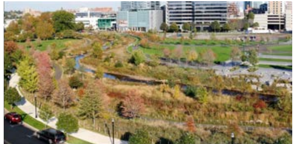
Mill River Park and Greenway an exciting ecological restoration in Stamford, CT
