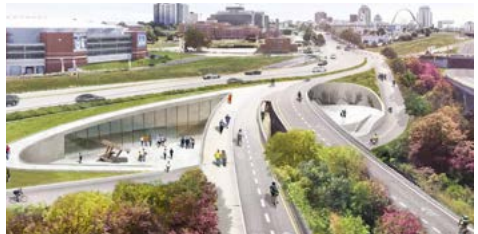
The Green Rivers Greenway St. Louis, MO, showing access, separation and planted areas for drainage.
