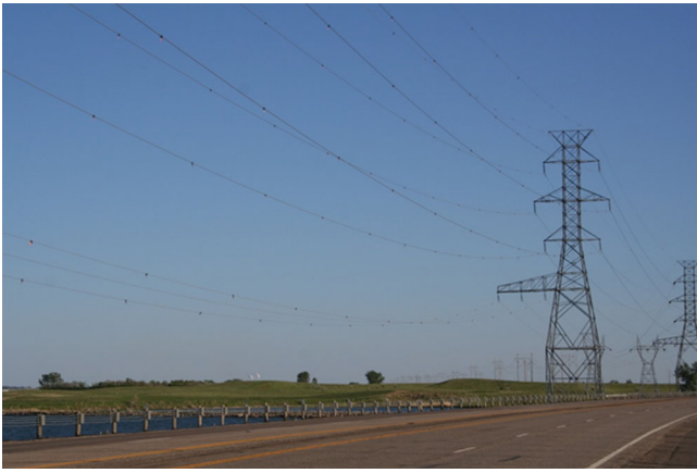
Figure 2. Line marking on non-energized overhead static lines (top 2 wires), energized transmission lines (center 6 wires), and energized sub-transmission lines (bottom 3 wires) during study of avian collision with power lines conducted from 2006 to 2008 in central North Dakota, USA.
